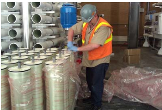
RO Vessel Installation
