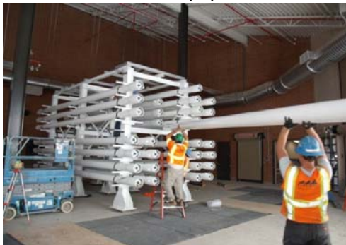
RO Vessel Installation
