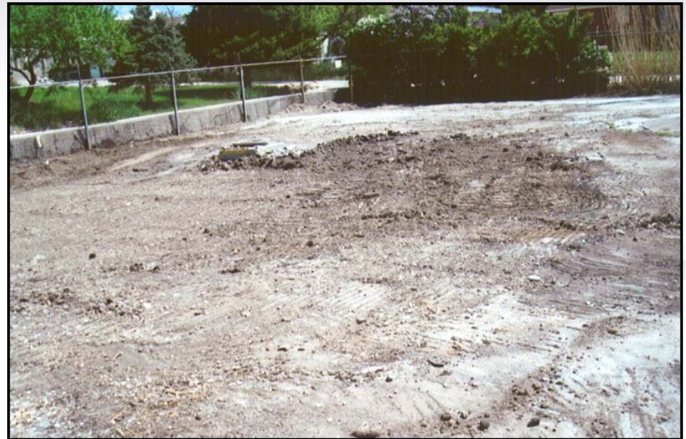
After well house demolition.
