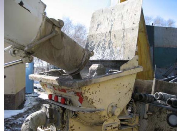
Installation of cement well seal
