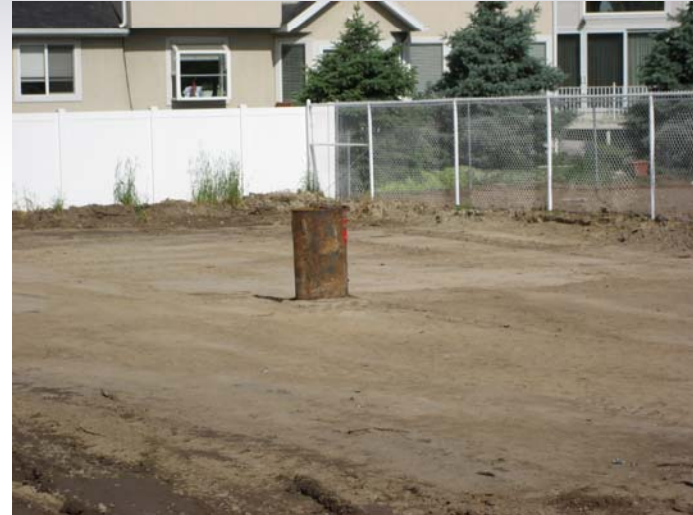
Completed Well at 987 East 7800 South 5 cfs capacity
