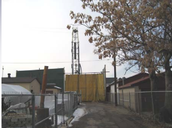
Drilling with reverse rotary rig
