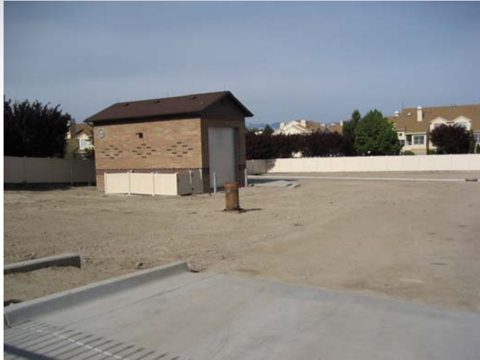
Completed Well at 7618 South 700 East 3.5 cfs capacity
