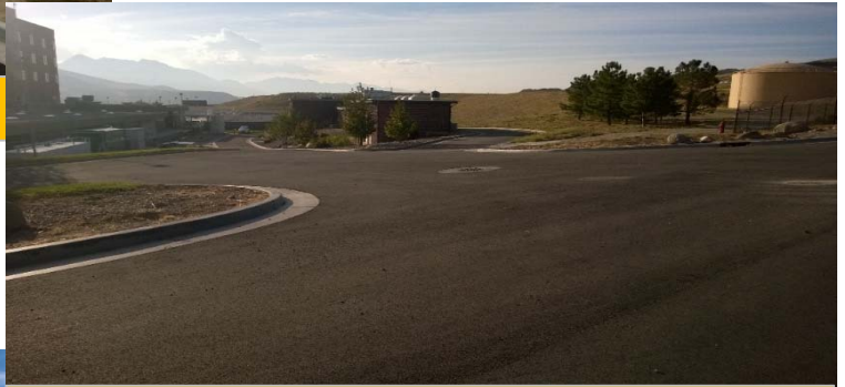
New Approach into JWTP
