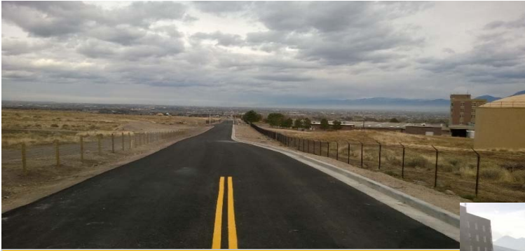
3200 West Access Road from MVC
