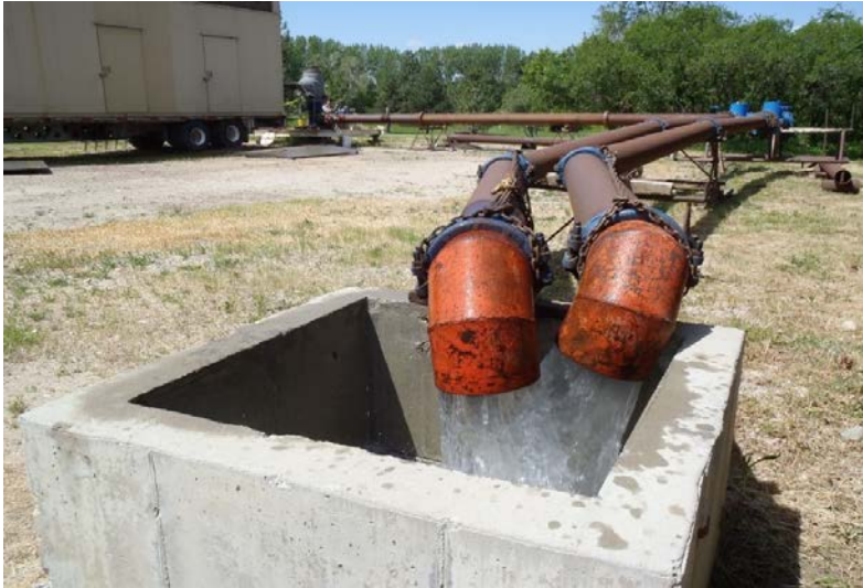
Etienne Way Well testing water discharge
