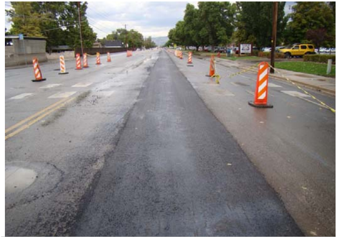
Asphalt trench restoration
