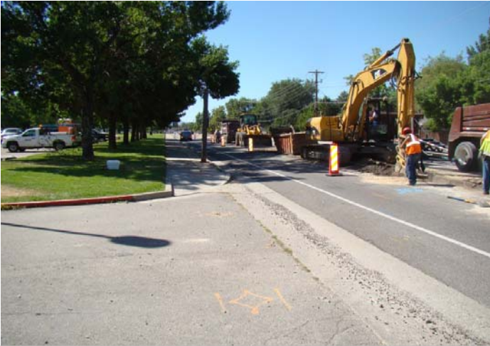
Pipeline construction on 1300 East near Cottonwood High School
