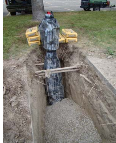
Typical fire hydrant assembly and installation
