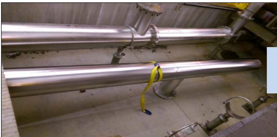
Installation of trench extension piping for new cartridge filter vessels
