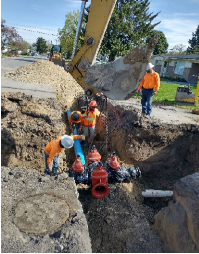
Installing new 4-valve cross in Murray
