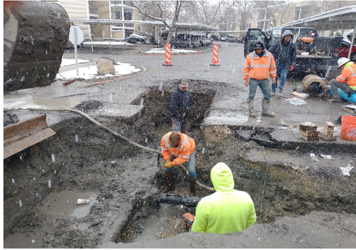
Demolition of old pipeline connection in Old Farm
