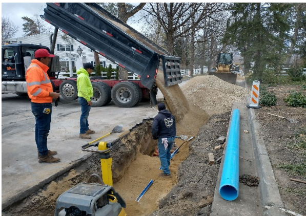
Backfilling pipeline in Old Farm
