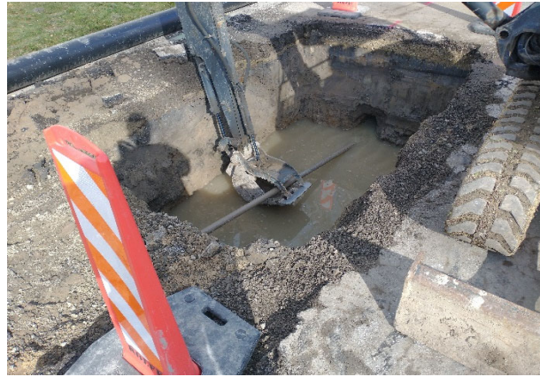
Drilling under creek in Old Farm
