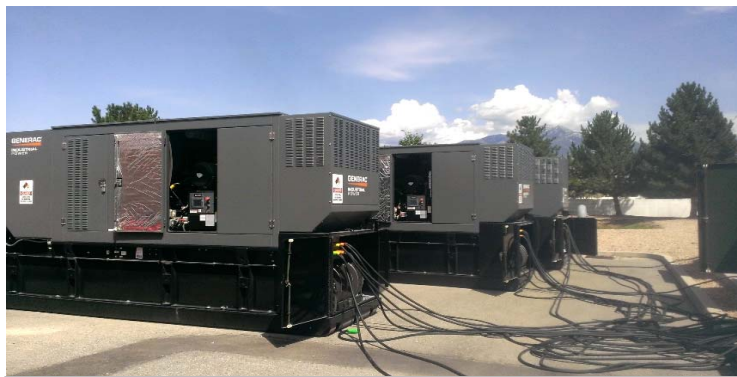
Staff training for cabling mobilization at 13387 South 3300 West
