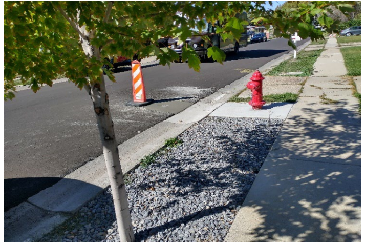
New fire hydrant, valve collar, and road asphalt
