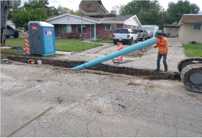
Laying new 8" PVC Waterline
