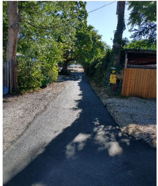
New asphalt over waterline trench
