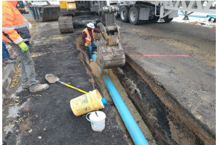
Backfilling new pipeline in trench
