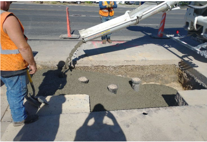
Pouring concrete around new mainline valves
