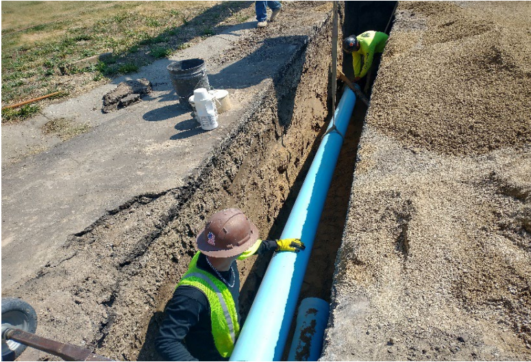
Laying new 8" PVC pipe
