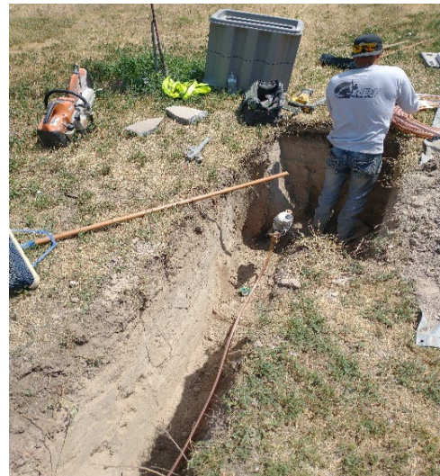
New setter installed in yard
