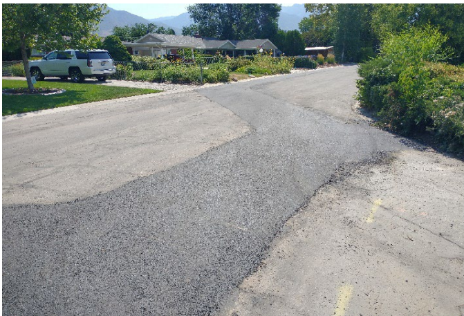
New asphalt over new pipeline
