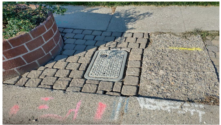
Completed new service connection box
