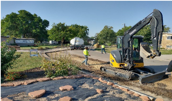
Compacting on top of new waterline
