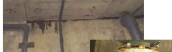
SW Corner Roof (must sawcut center)
